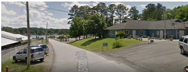
Commission on Aging Building
